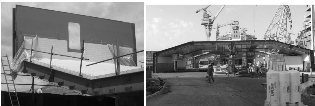
Fig.6 Shelter decks insulation before mounting
