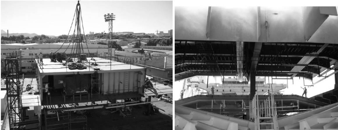
Fig.8 Hull block Shelter deck/deckhouse instalation
