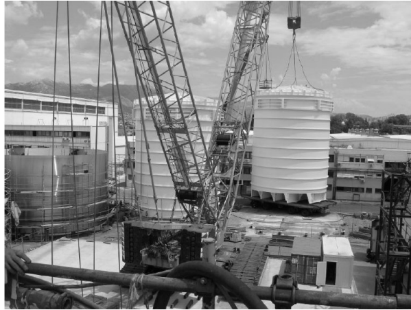
Fig.16 Cargo tanks instalation
