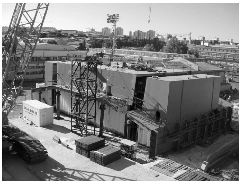
Fig.7 Three hull blocks Shelter deck/deckhouse
