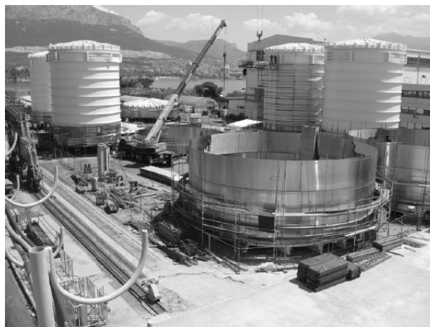
Fig.15 Cargo tanks building area in shipyard
