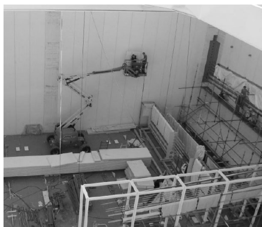
Fig.5. Cargo space insulation
